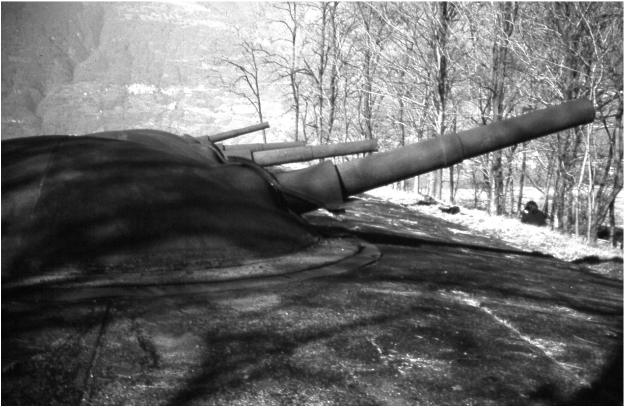
Fort Montecchio Nord, in Colico (Lecco). The only Italian First World War fort to survive intact. In the foreground is one of the four revolving turrets ("S" installation, Schneider), armed with a 149/35 cannon (photo G. Padovan).
